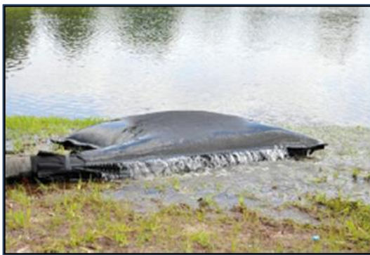
Plate 3-2 Silt Bag with water being pumped through.
