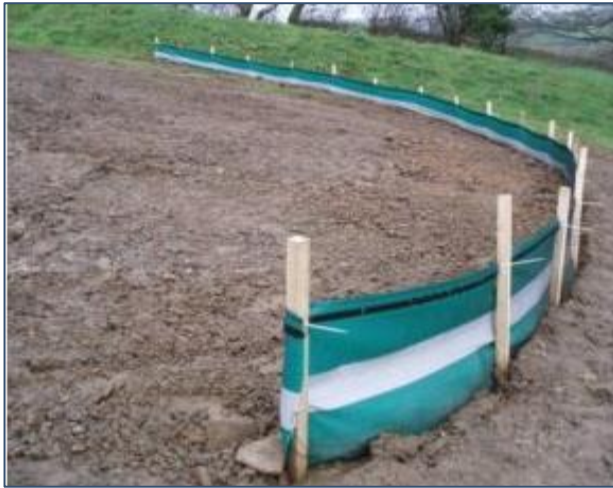
Plate 3-1 Embedded Silt Fence
