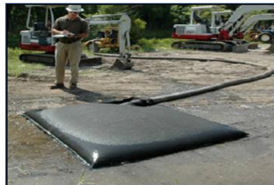
Plate 3-3 Silt Bag under inspection.
